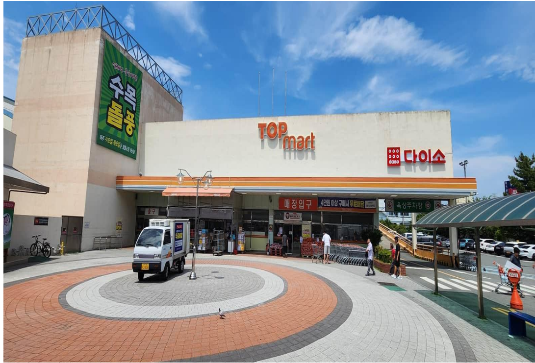
Parking Lot Waterproofing Top Mart Geumsa Branch, Busan
