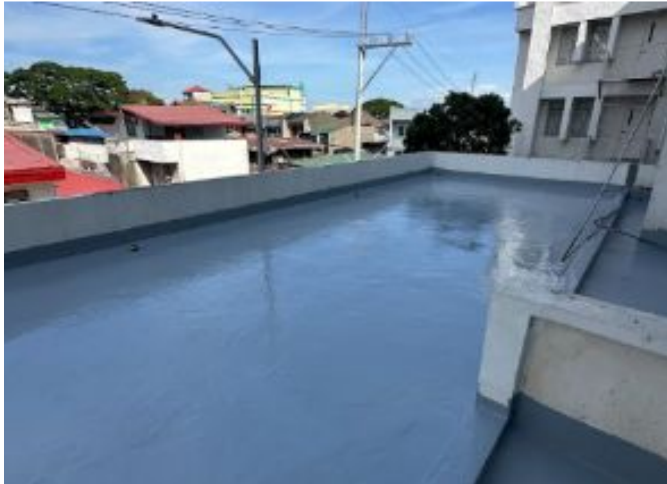
ANTIPOLO CITY HALL - 3RD FLOOR ASSESSORS BALCONY
